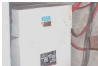
Installation of Capacitors
