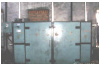
Steam line Modification (Electrical Heating Eliminated)
