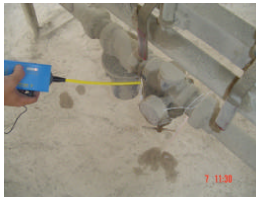
Figure 2: Sound leak detector method
