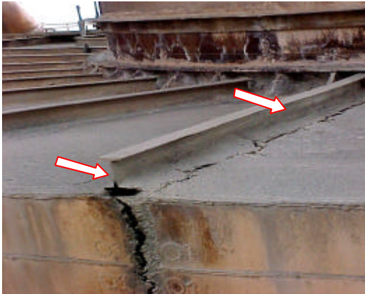
Figure 2: Leaks source at cyclone pre-heater; cyclone roof is opened
