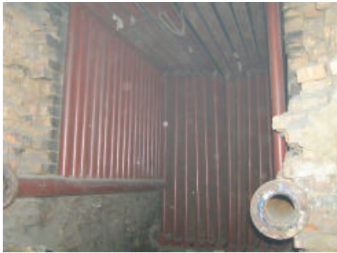
Figure 1a: Installation of new bent-tubes
