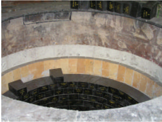
Figure 1 Insulation improvement of Ladles
