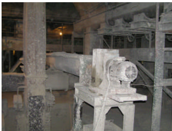
Figure 1. One of the installed motors for rehabilitated strew conveyers
