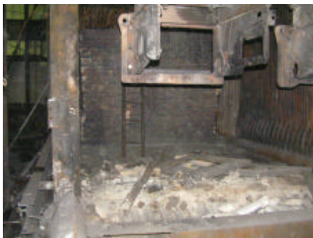
Figure 1. Reconstruction work for district heating boilers
