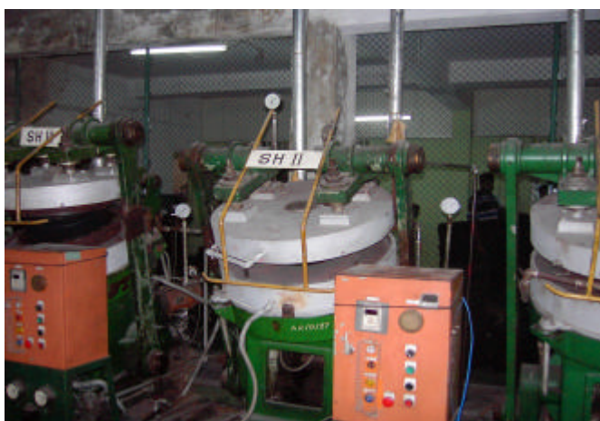
Figure 1: Un-insulated moulds at RPD at AMW
