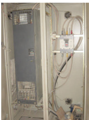
Figure.1 The VSD installed on motor of FD Blower of Kiln 1
