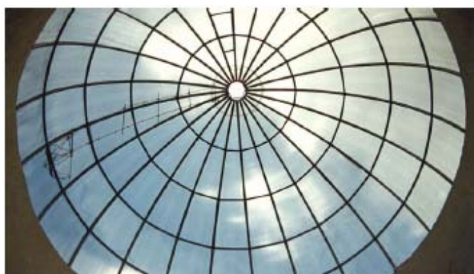
Figure 14. Atrium with FRP dome
