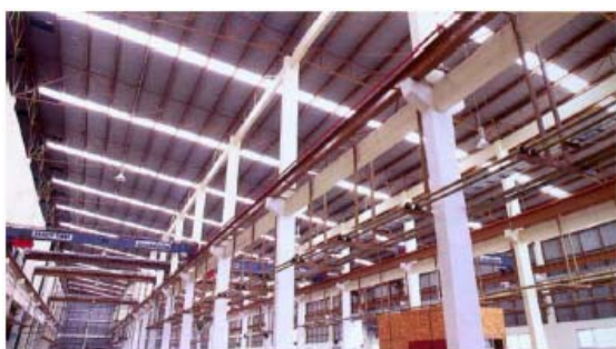
Figure 13. Day lighting with poly carbonated sheets
